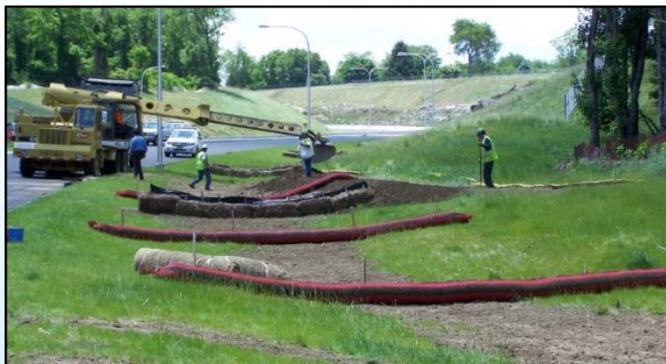
Compost filter socks used as check dams to control runoff
